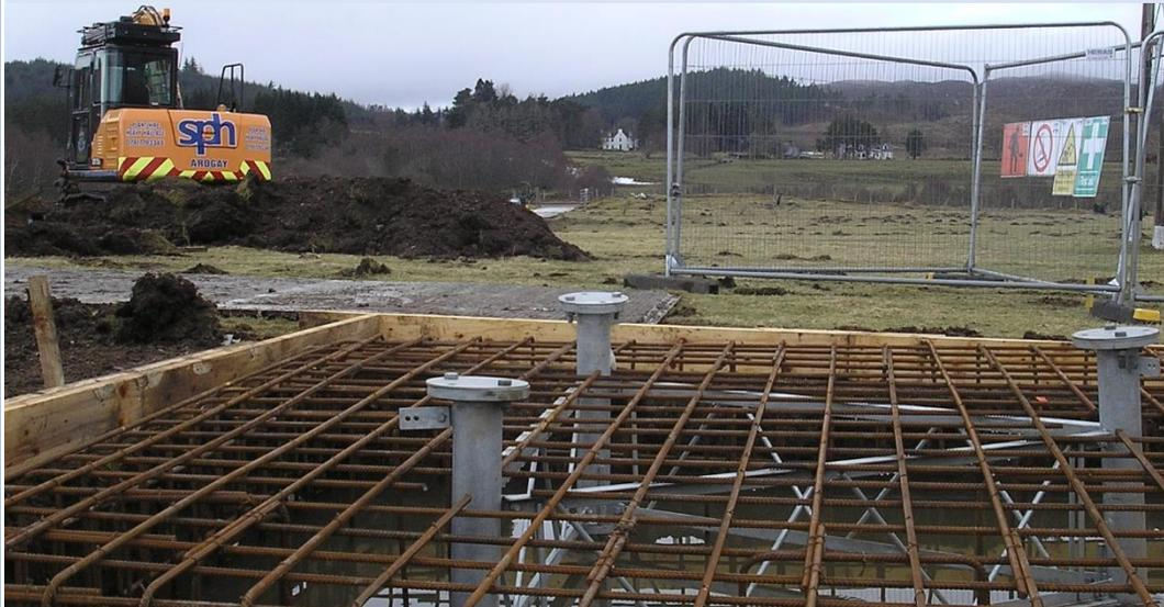
A New Mobile Phone Mast is now being installed near Whitebridge for telecoms firm EE. The lattice mast will have three legs and be 30 metres in height. It is located on Garrogie Estate ground close to the B862 about 190 metres above sea level. Mark Shaw of contractors SPH from Ardgay who are installing the foundation pad for the mast said 'This mast will bring 4G signal to a very wide area and not just Whitebridge and Lochgarthside.' Dell Lodge is visible in the photo above.
